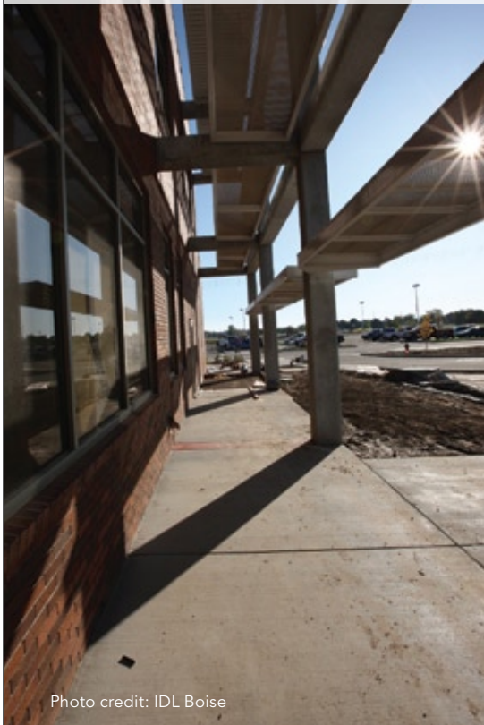
External shading at south façade along east classroom wing
