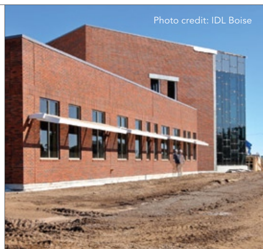
View of south façade at faculty offices in west wing
